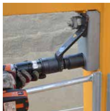
Assembly of taper pin connection with battery nut runner
