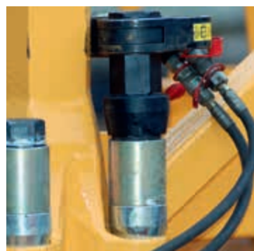
Tower section assembly with FSX
